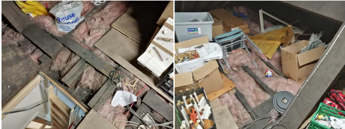
Figure 1 - Condition of existing loft insulation.
